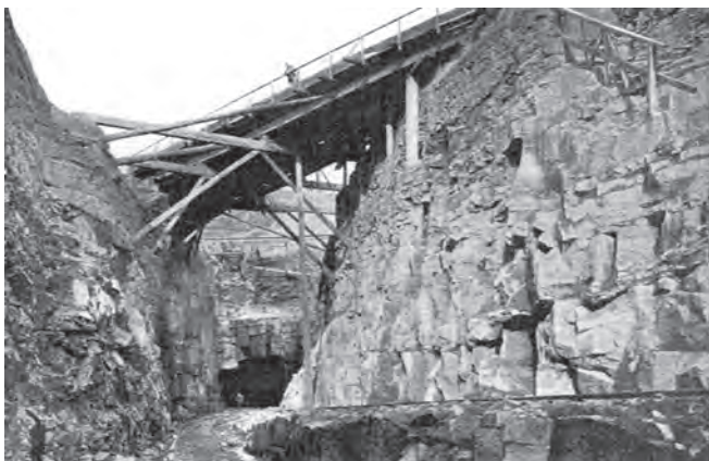
The southern entrance to the Queensbury tunnel during construction
